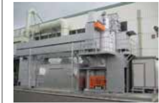
Deodorizing equipment (Kyushu factory)
