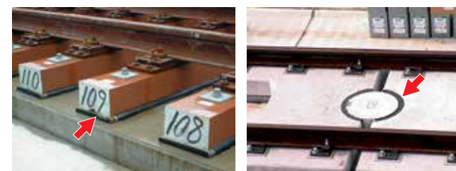
Lining material for railway tracks
